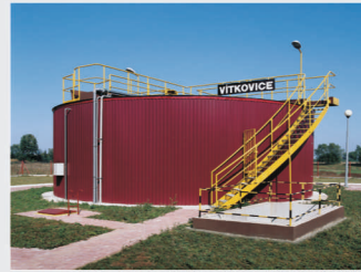
Waste water treatment plant, Poland Realization: 1998 Location: Radymno Capacity: 1 500 PE
