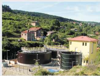
Waste water treatment plant Bulgaria Realization: 2013 Location: Jablanica Capacity: 5 000 PE Purpose: Complete delivery wastewater treatment plant Model: HYDROVIT®P
