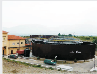
Waste water treatment plant Bulgaria Realization: 2000 Location: Sopot Capacity: 25 000 PE Purpose: Complete delivery wastewater treatment plant Model: HYDROVIT®P
