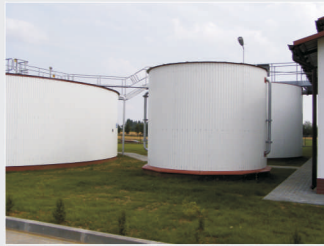
Waste water treatment plant, Poland Realization: 2015 Location: Wierzawica Capacity: 16 000 PE Purpose: Complete delivery wastewater treatment plant Model: 2x HYDROVIT®SI 400, 1x 2x HYDROVIT®SI 800
