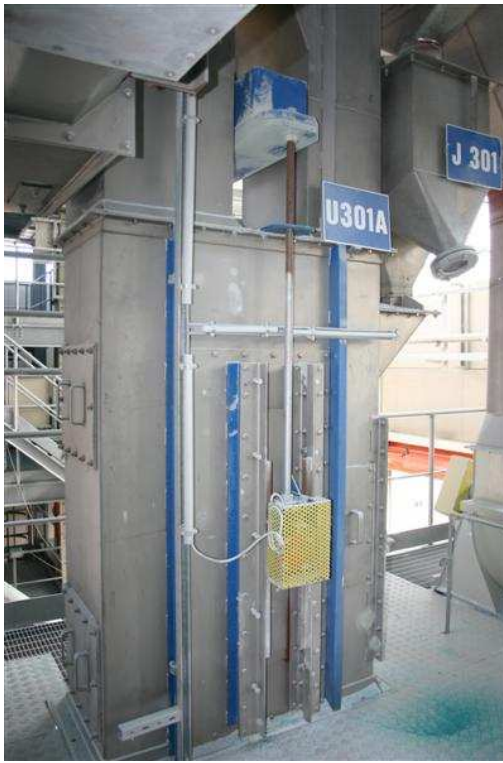
Samec Bucket Elevator ET 1000x600 – tension station
