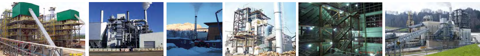
✓ 77 MW hot gas generator with 25 MW thermal oil heater in membrane wall design
